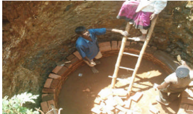
(4) The pit of one of the biogas plants being prepared
